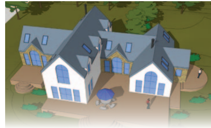
New build, Co. Waterford • Off-site timber frame. • Air-to-water, solar, heat recovery.
